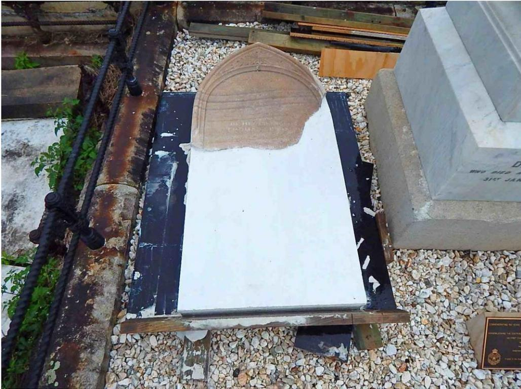
The repaired Brown/Seymour headstone. The white portion is the concrete blank which was be placed in and secured to the existing footings. A plaque will be affixed to the bottom of the exposed concrete.
